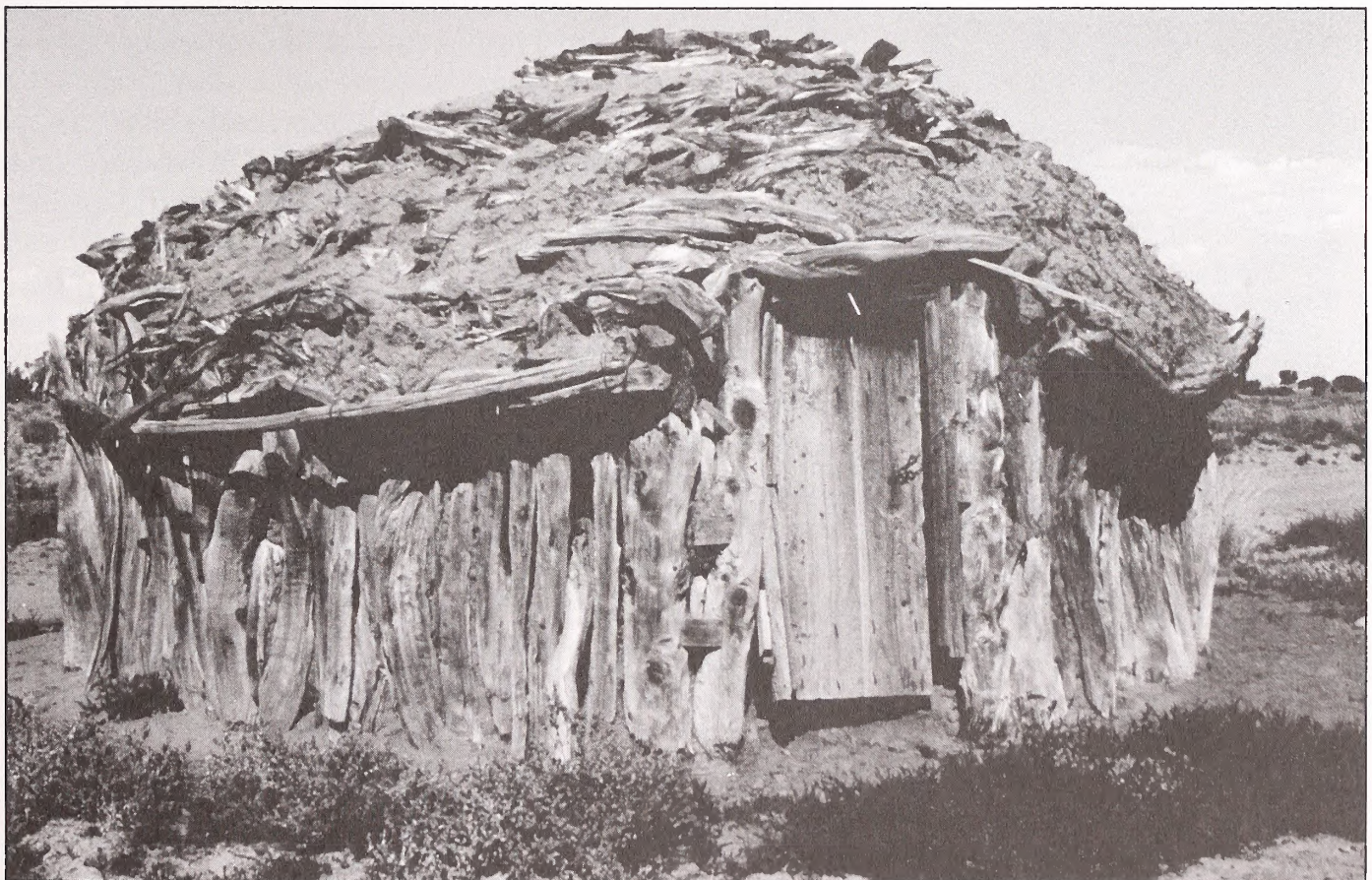
A hogan made from wood. The traditional Navajo home always had a door facing east.
